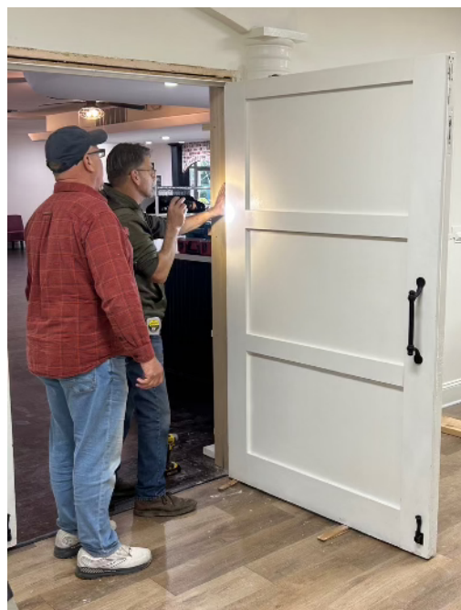
Ron Pane, left, and Matt Longo inspect a sagging door into the Venetian Room. Volunteers took apart the door jamb and rebuilt it. They adjusted several other doors in the building as well.
