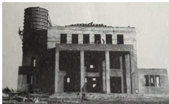
This post-World War II photo shows construction well underway on the new St. Mary's Church in east Sacramento. The groundbreaking took place on Sept. 29, 1946, and the first Mass was offered on Aug. 1, 1948.
