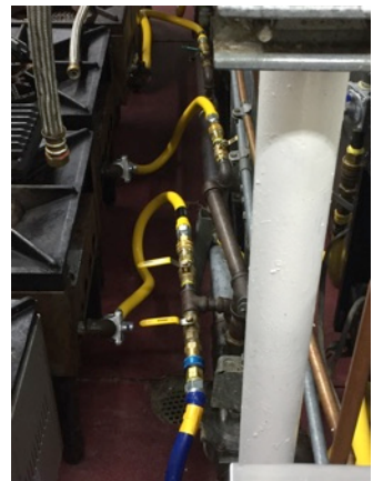
Newly installed gas lines are among multiple improvements that have been made in the Dante Club kitchen.
