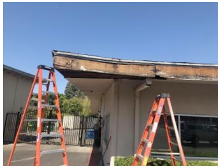
Workers repair a fascia on a portion of the building as part of the Dante Club's recent renovation effort.
